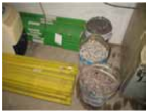
The "Good" - welding control
